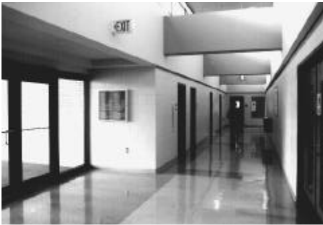
The renovated north hallway with its new central entrance on Dickson Street. The Physics Library is to the right and Physics Office is at the far end.
