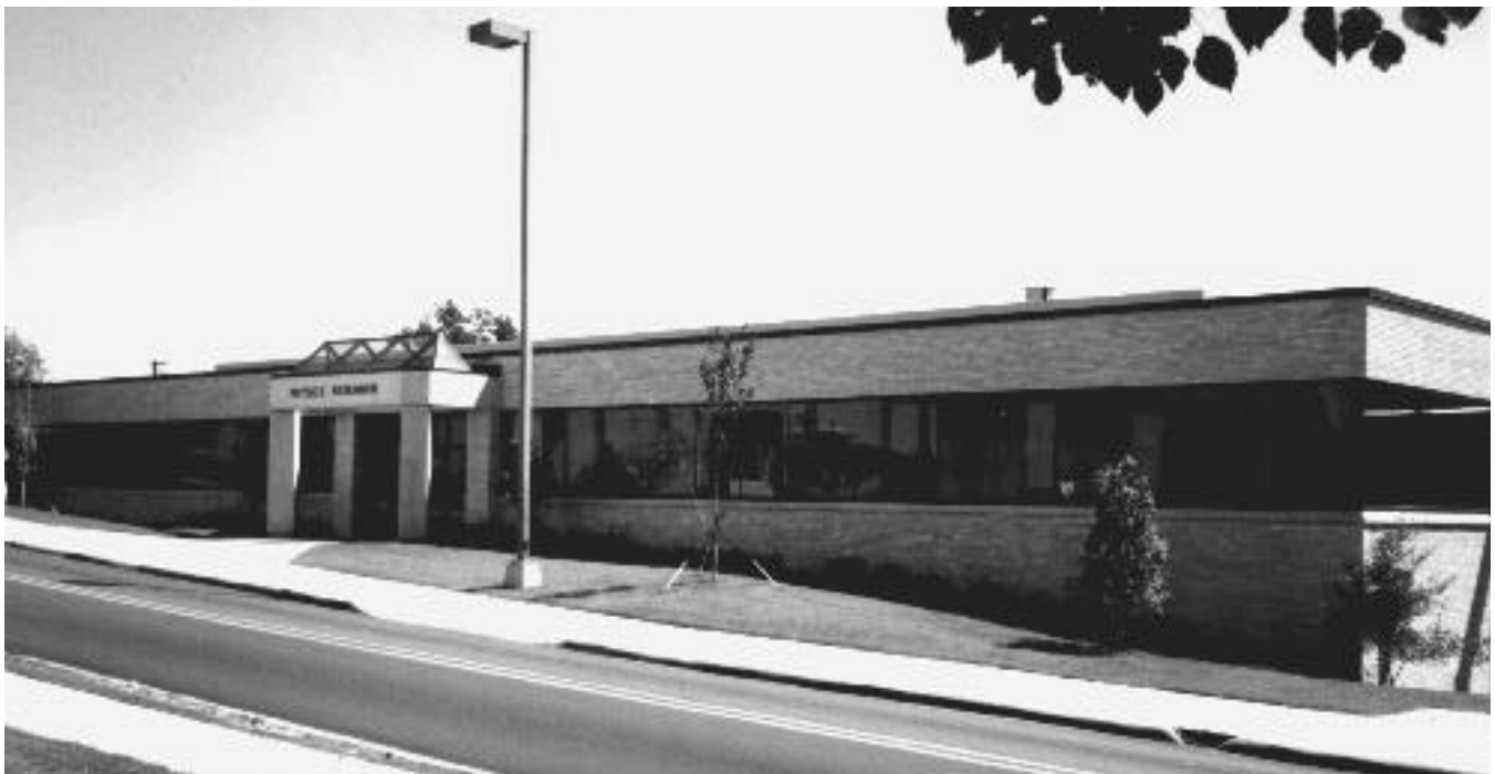
Front view of the renovated Physics Building. Dickson Street is in the foreground.
