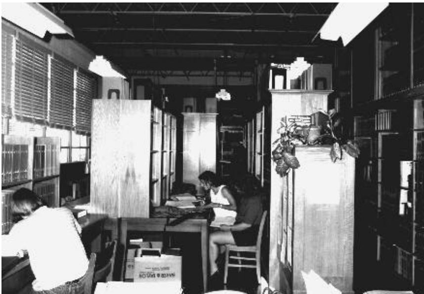
A view of the Physics Library before the renovation. The library had totally outgrown the space and looked like a book warehouse with journals stacked to the ceiling and very little seating space. Ceiling open to fiberglass roof insulation and warehouse lighting connected by extension cords can also be seen.
