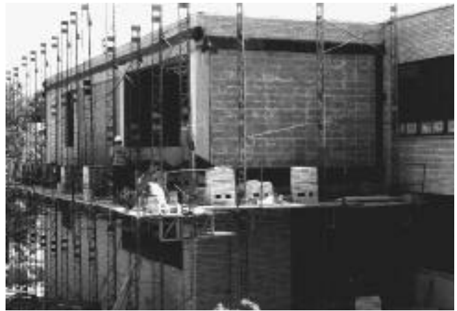
The new wing under construction.
