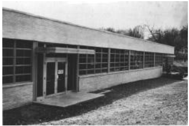
Front of new Physics Building facing Dickson Street. This building was completed in June of 1952
