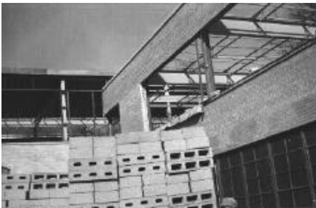
Building under construction in 1951 showing hadite block and brick walls.
